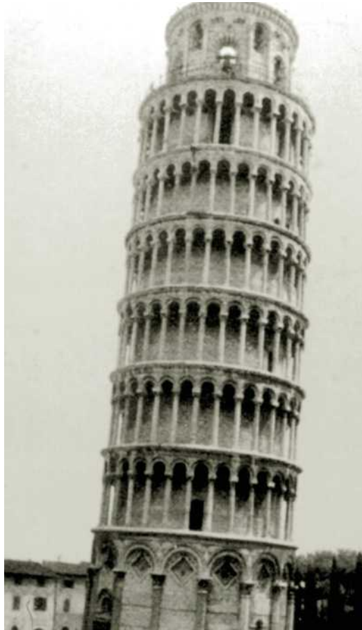
Figure 1.2 Leaning Tower of Pisa, Italy (Courtesy of Braja M. Das, Henderson, Nevada)
